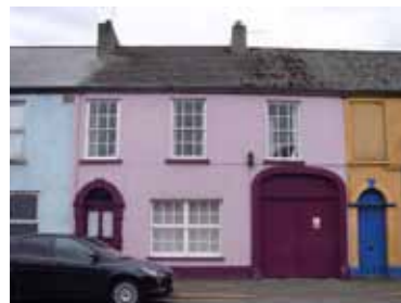
Coloured and painted render building frontages
