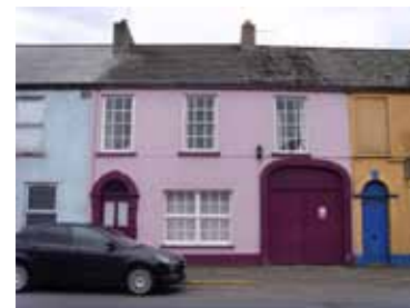
Coloured and painted render on building frontages
