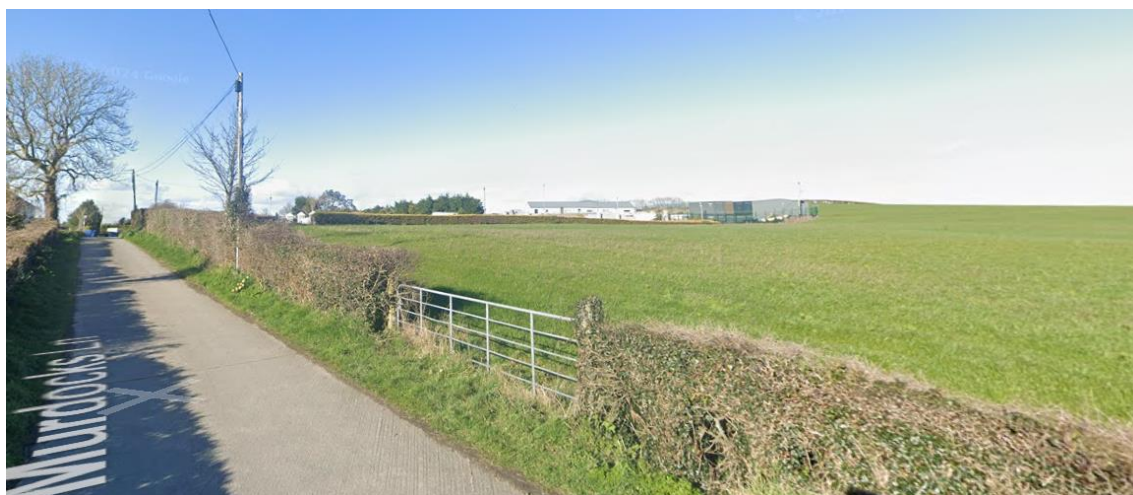
Figure 12: View of site from Murdock's Lane
