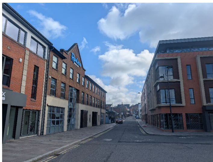
Photo 7: 4 Storey Building at corner of Hibernia Street (RHS)
