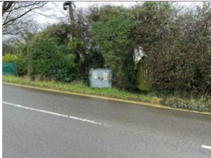
Figure B6 – Existing Kiosk
