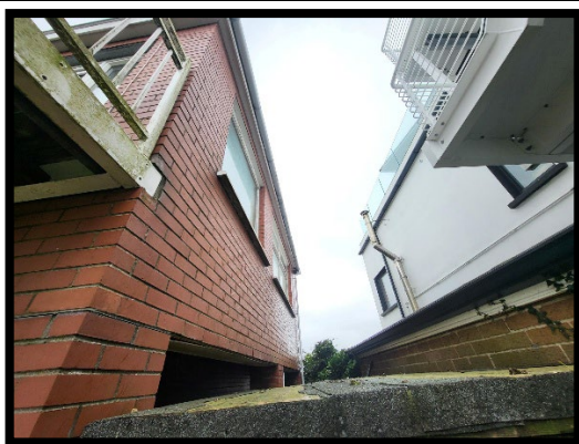
Existing south elevation of dwelling.
