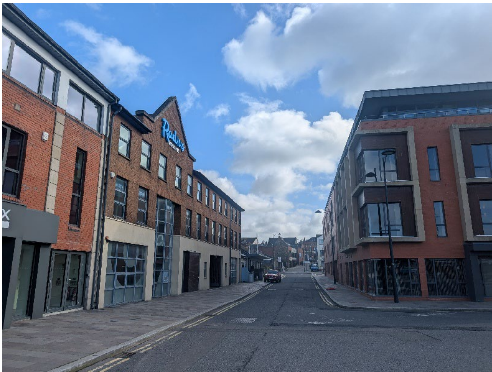
Photo 7: 4 Storey Building at corner of Hibernia Street (right of photo)
