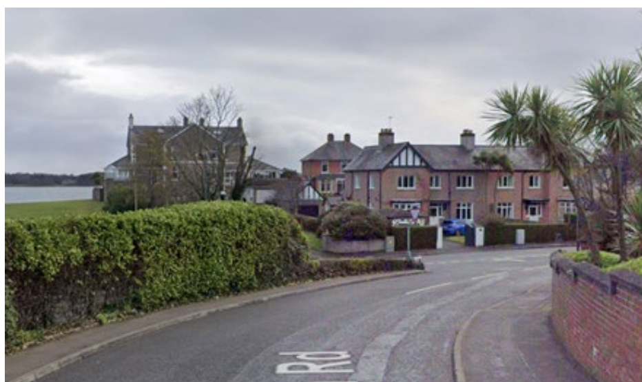
Fig 11 – View of existing dwelling from Clifton Road
