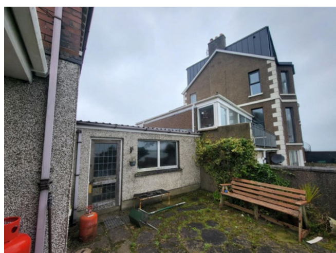
Fig 3 – Large dormer extension to No. 82
