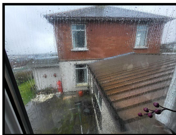
View from window of no.82.
