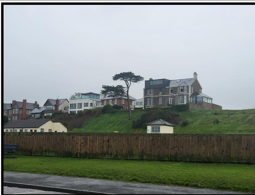
Fig 2 – View of site from Seacliff Road
