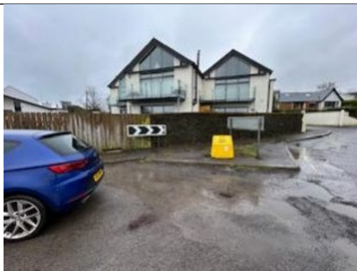
Figure B1 – view of site, taken facing south
