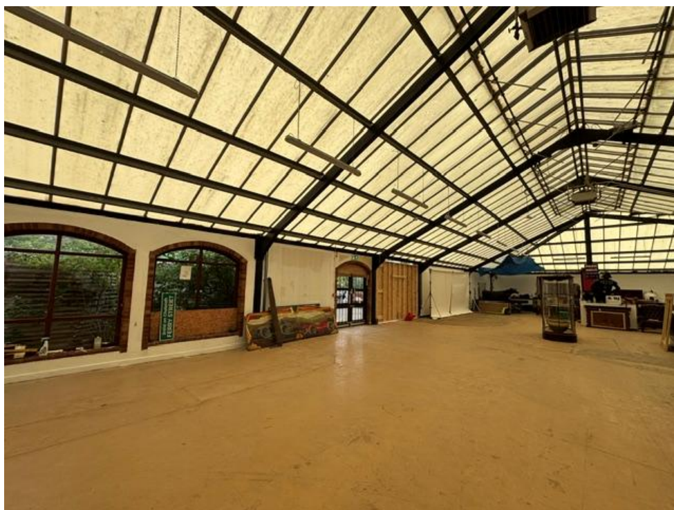
Internal of existing building formally used as Dickson's Garden Centre
