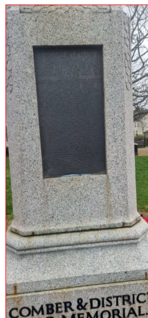
Photo of Existing
