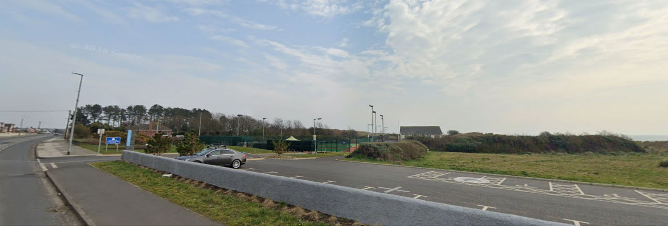
APPROACH FROM THE SOUTHWEST
