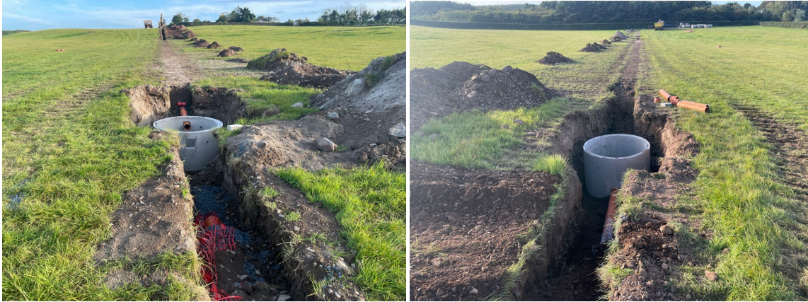
Fig 4. MH16 and MH17 during installation
