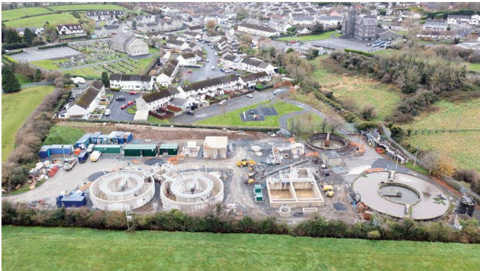
Ballygowan WwTW under construction (December 2021) – Courtesy of NI Water
