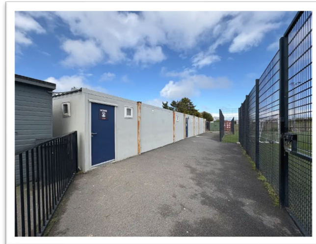
Existing changing room facilities between service yard and smaller pitch to be extended
