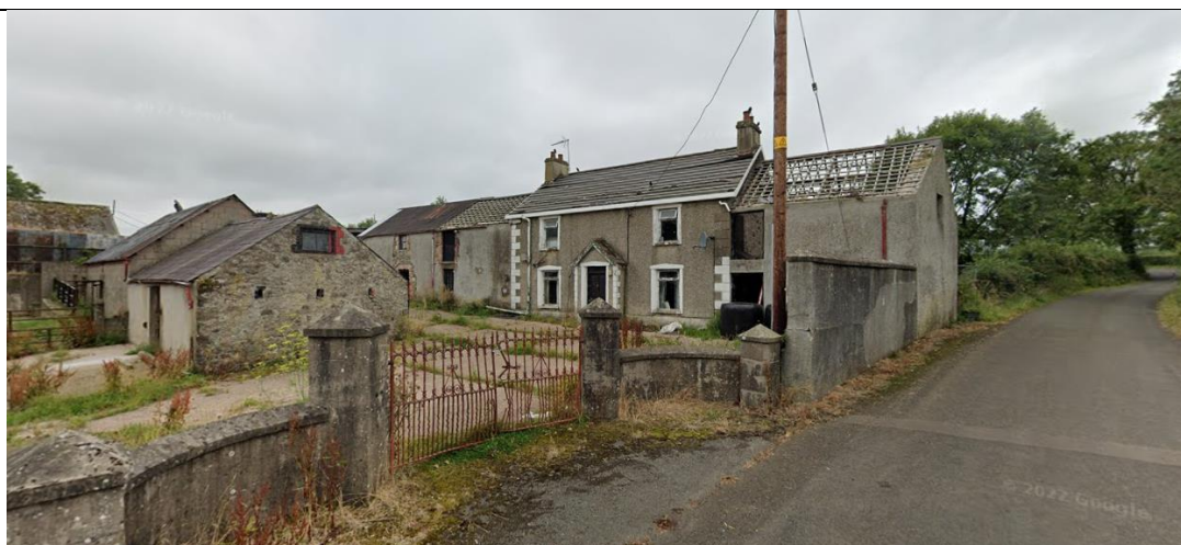
Figure 6: Google street view image of 65 Rathmore Road. – Appeal reference 2018/A0031
