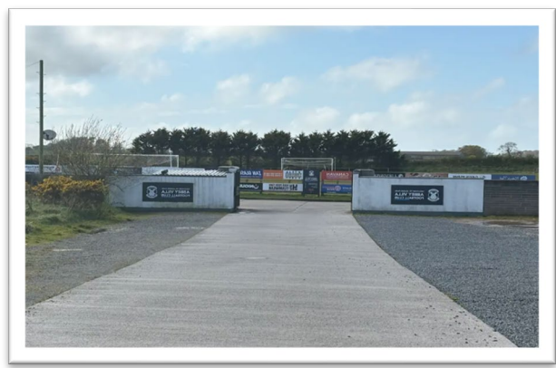
Gated Entrance into Football grounds
