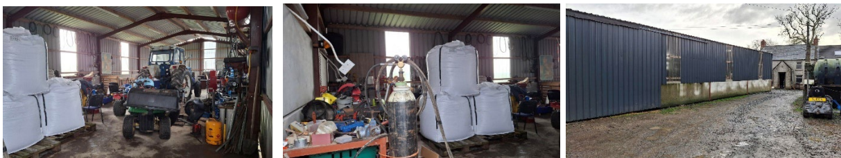
Figure 7 Photographs showing the use of one of the shed recently granted permission in 2023.
