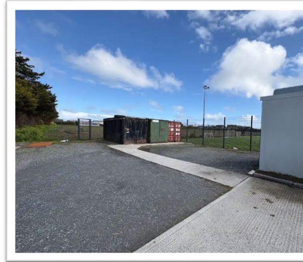
View from eastern extent of service yard towards small pitch to be extended
