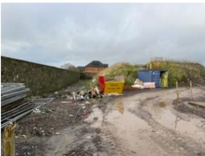
Figure A4 – southwestern corner of site
