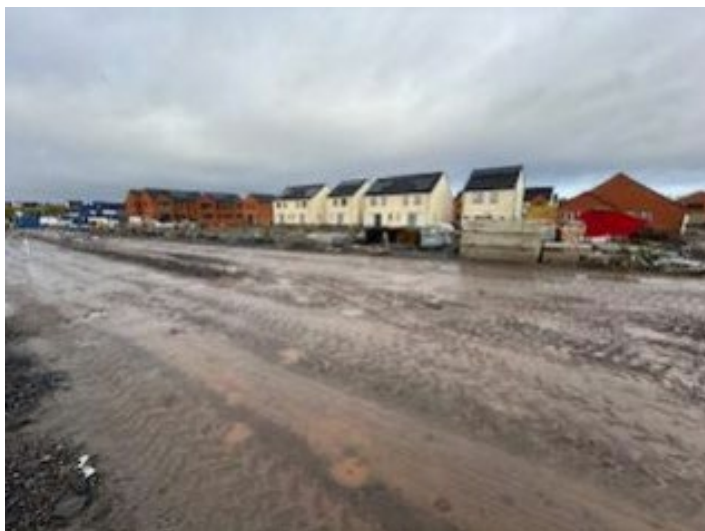
Figure A2 – View northwest from site entrance
