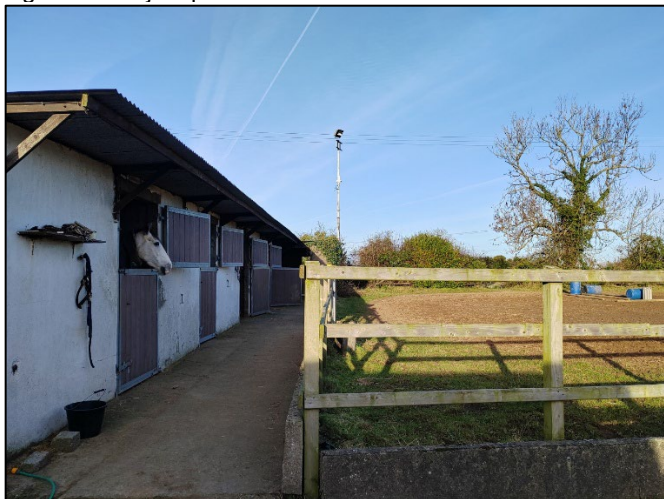
Figure 4. Subject pole with the CCTV cameras
