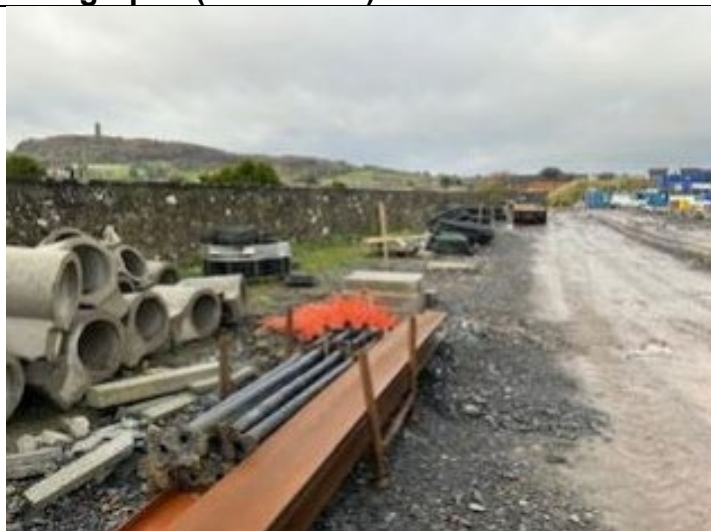
Figure A1 – View west from site entrance
