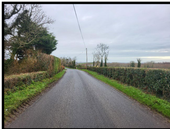
Figure 9 - View on approach from south
