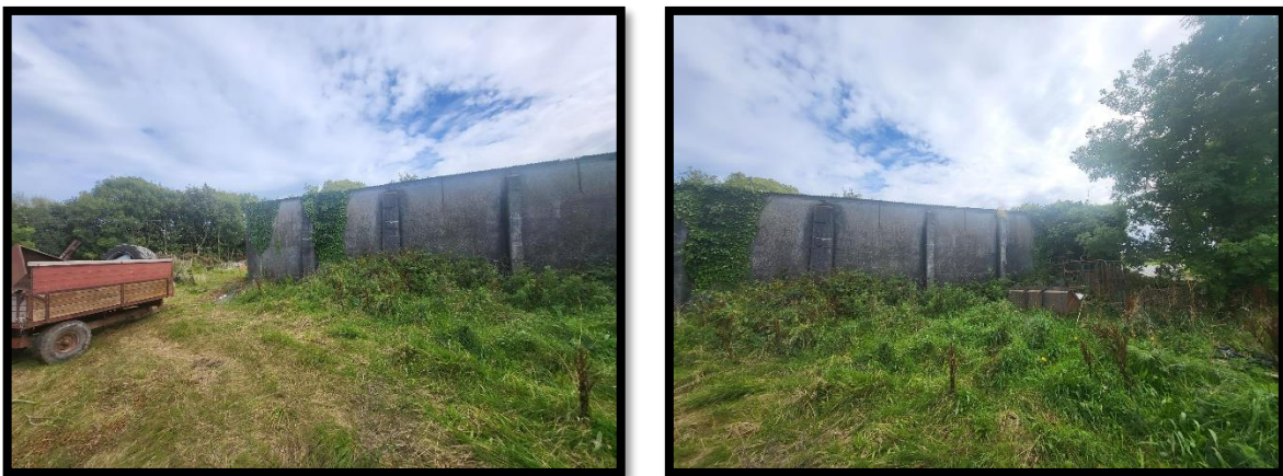
Figure 4: Photos of the extended part of the building
