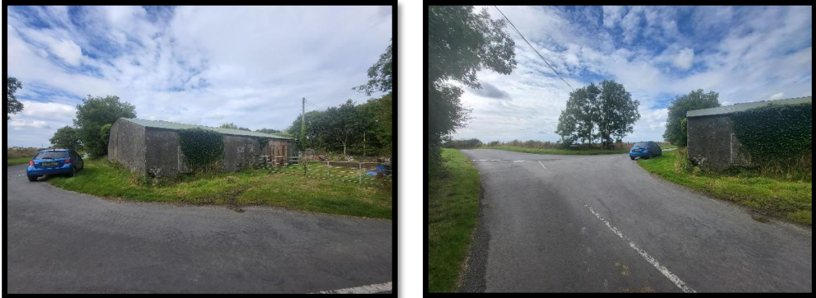
Figure 3: Photos of original section of the building
