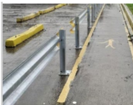
Figure 1 Example of physical barrier and a separated walkway
