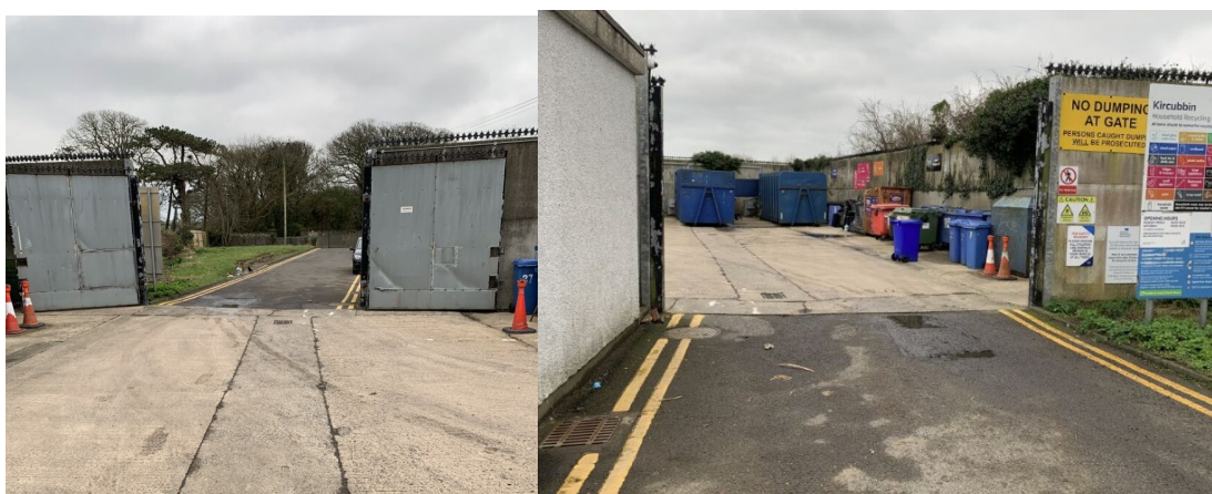
Figure 7 Kircubbin HRC entrance and signage
