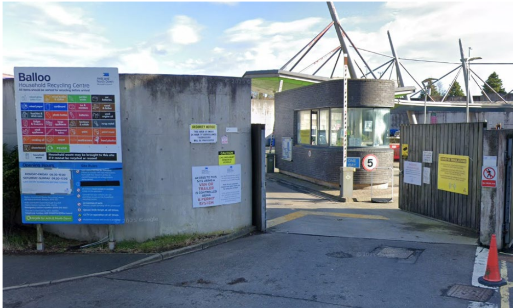
Figure 3 Balloo HRC entrance and signage
