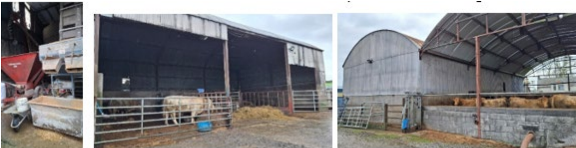
Figure D. Photos showing the existing buildings used to house cattle and the meal preparation station.
