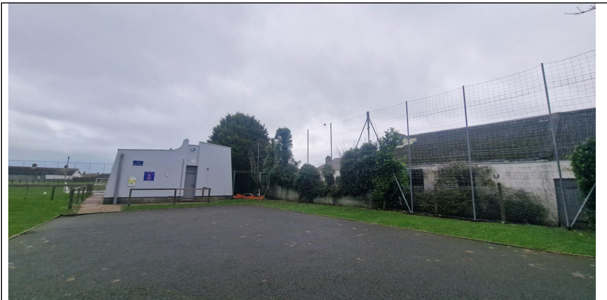
Existing pavilion building and boundary with No. 8
