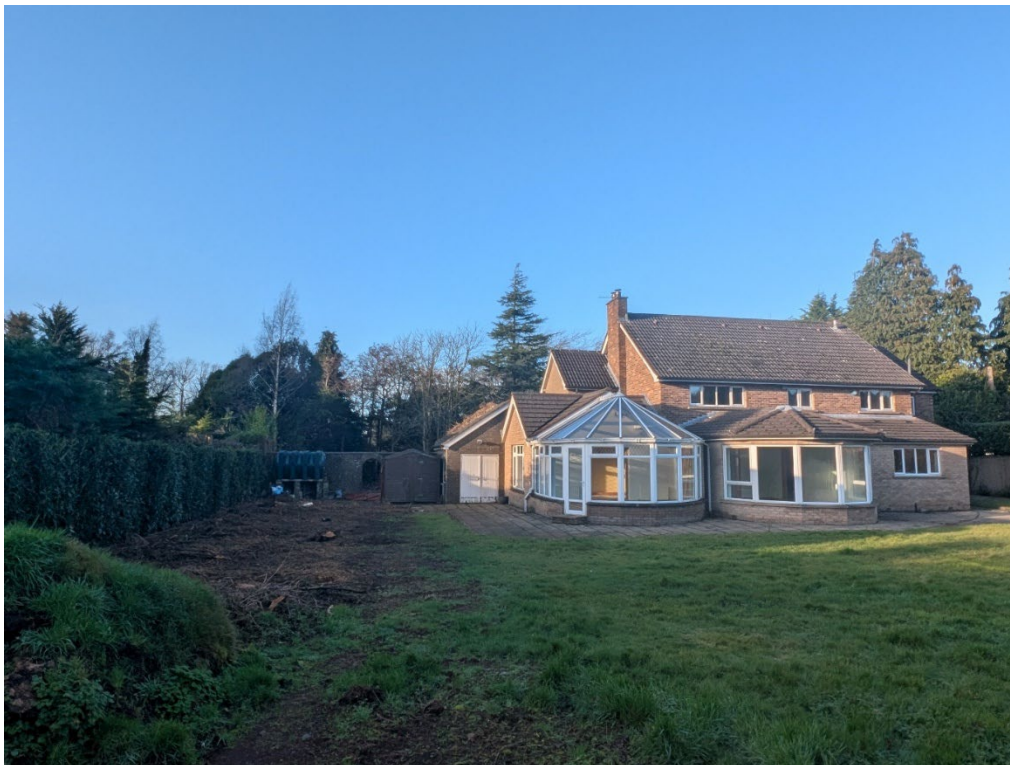
Photo 2 – Rear Elevation 31 Old Cultra Road
