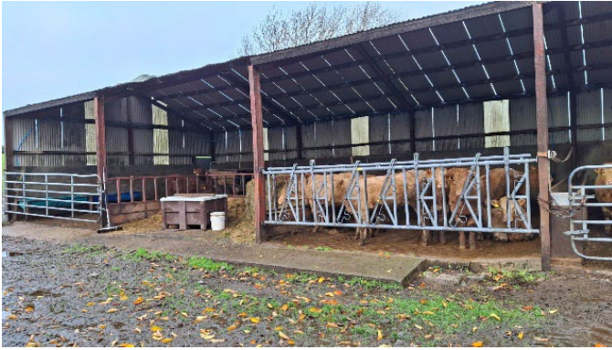
Figure C. Existing shed to the north of 15B Abbacy Road
