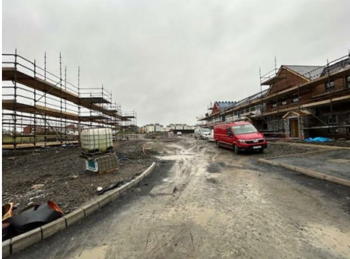
Figure A2 – Plots 14-19 under construction, with proposed siting of plots 20-23 beyond
