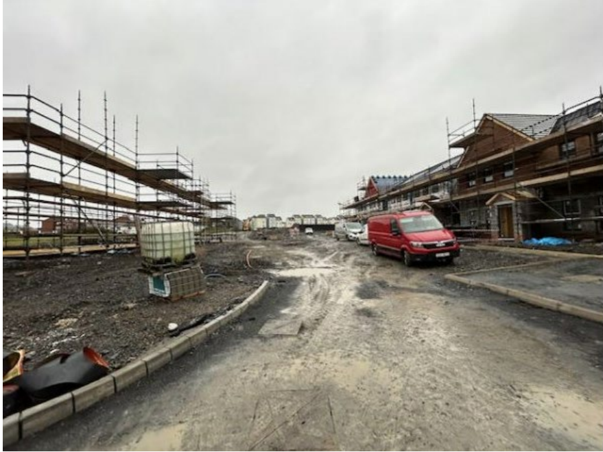
Figure 2 – plots 14-19 under construction, with proposed siting of plots 20-23 beyond
