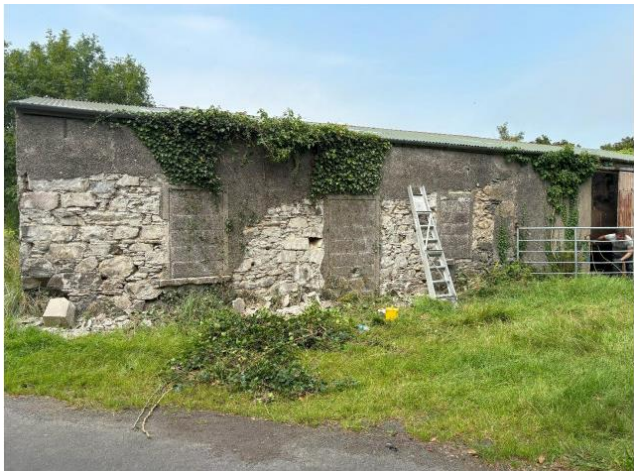
Figure 7: Photograph submitted by the agent to demonstrate removal of portions of render.
