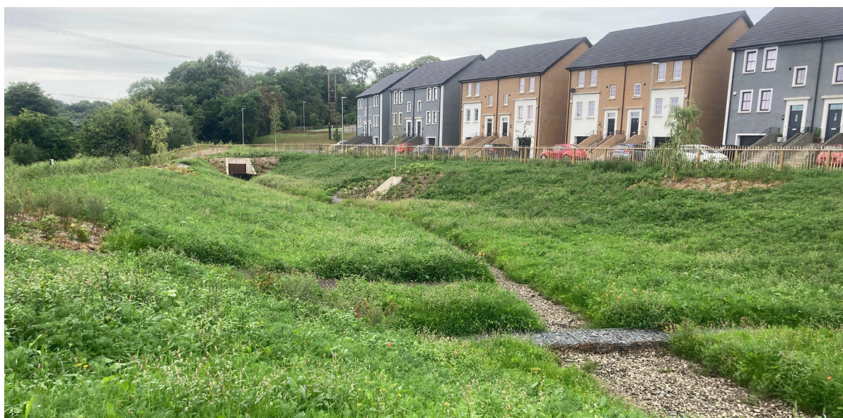
Large SuDS Detention Basin at Belmont Hall Drive
