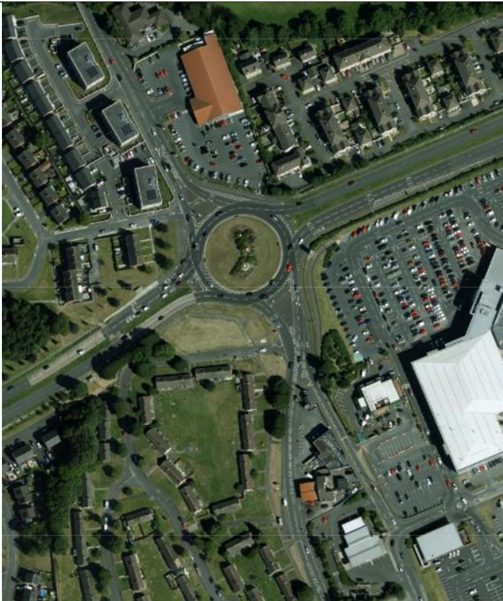
Figure 2 – Aerial View of Site and Surroundings
