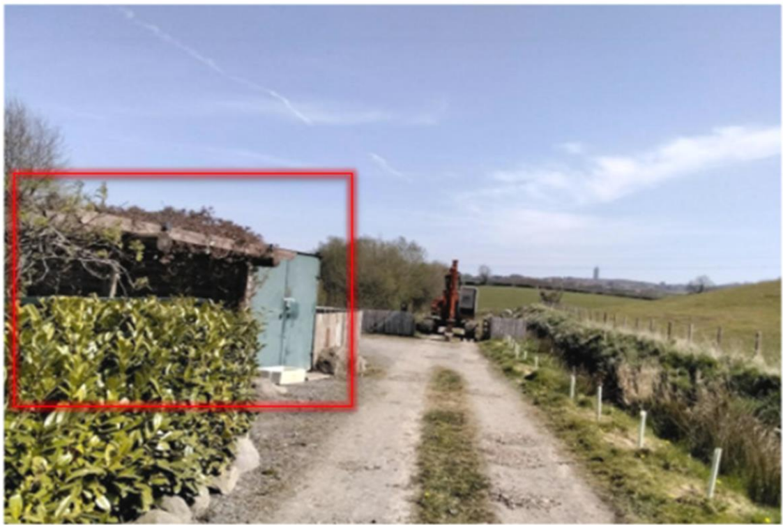
Photographs showing side of hide (in green) and wooden pergola on western elevation (April 2025)
