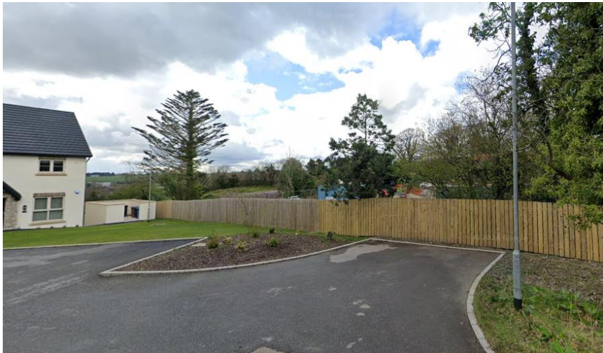
Figure 5 – View of site from new development at Tullynagardy Green
