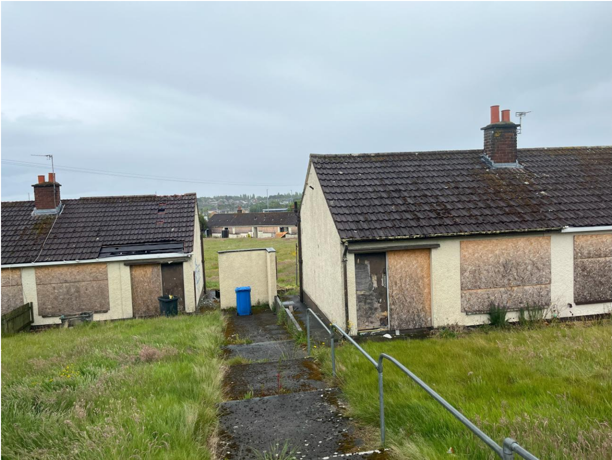
Photograph 6 – View between dwellings on Skipperstone Avenue towards central enclosed amenity area to the rear of dwellings
