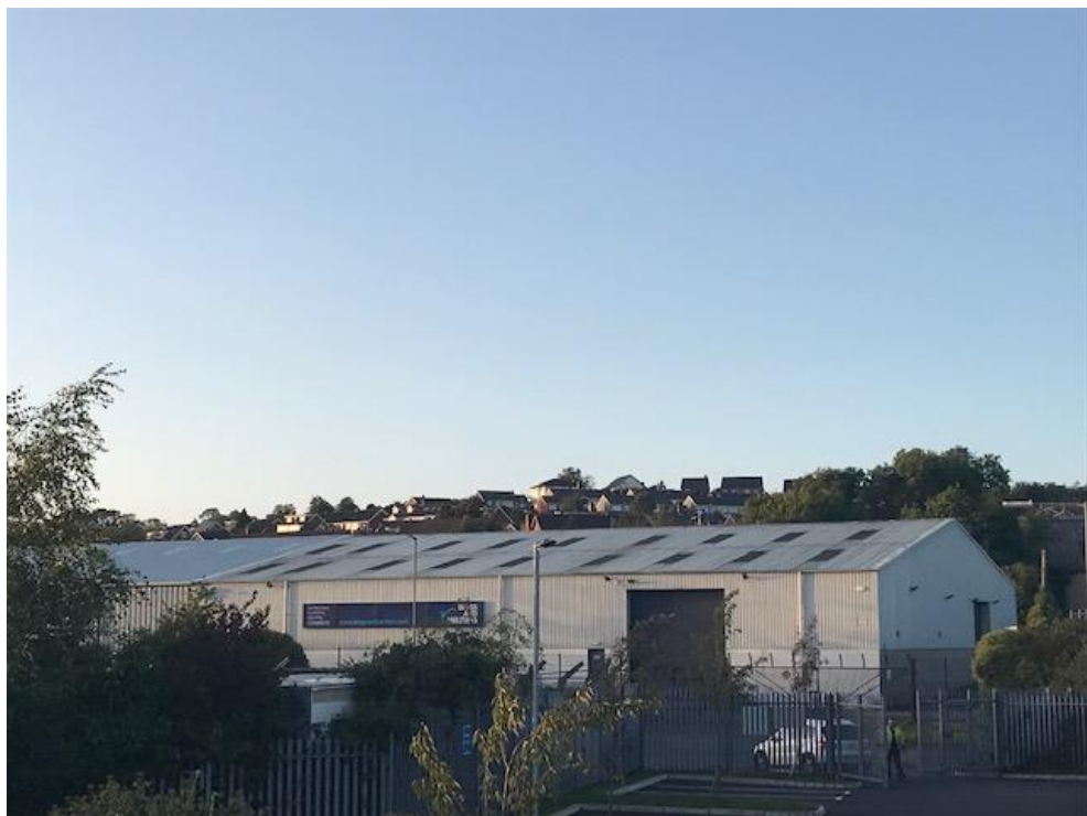
Figure 22 – View towards site from Hardford Link showing existing dwellings at Galla Way in skyline
