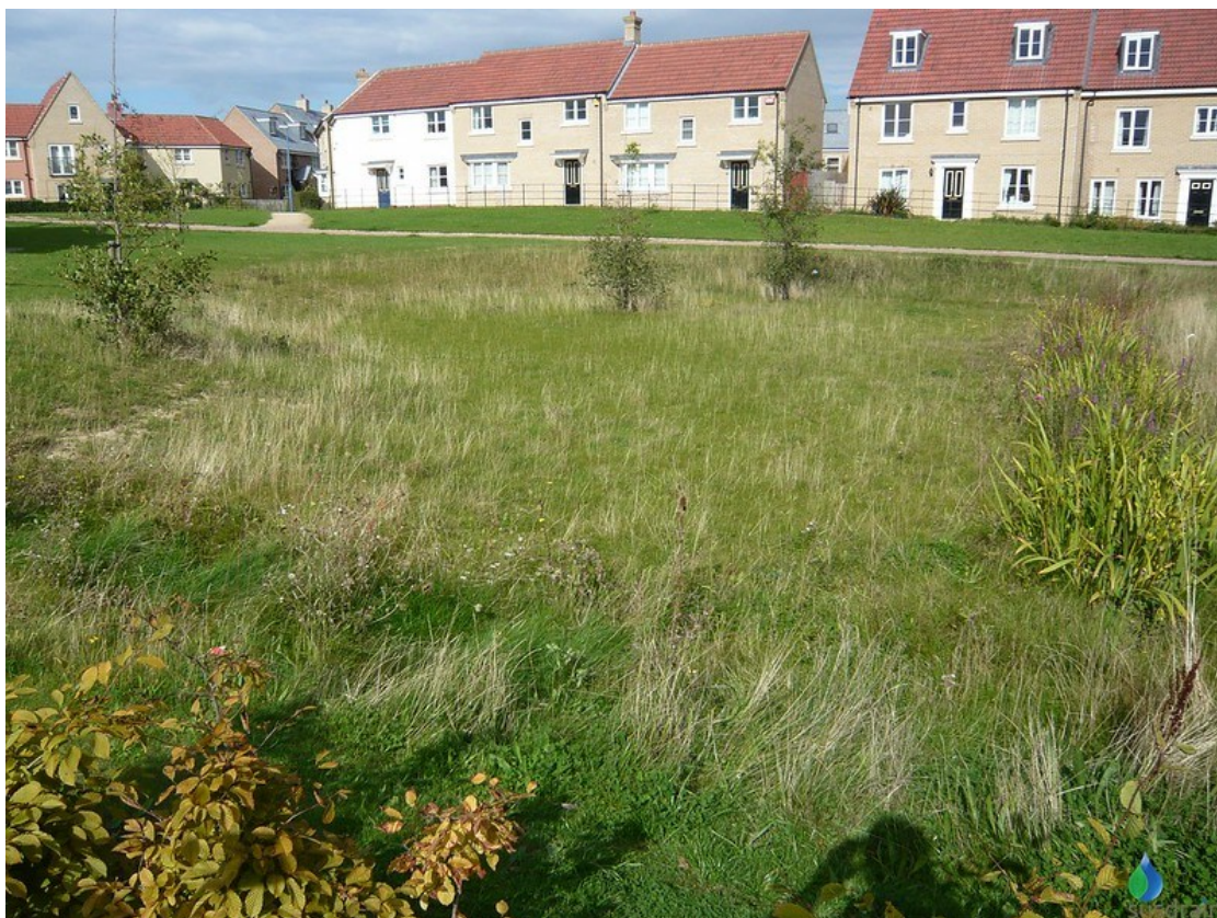
Figure 1: Detention Basin at Lamb Drove site , Source: Susdrain
