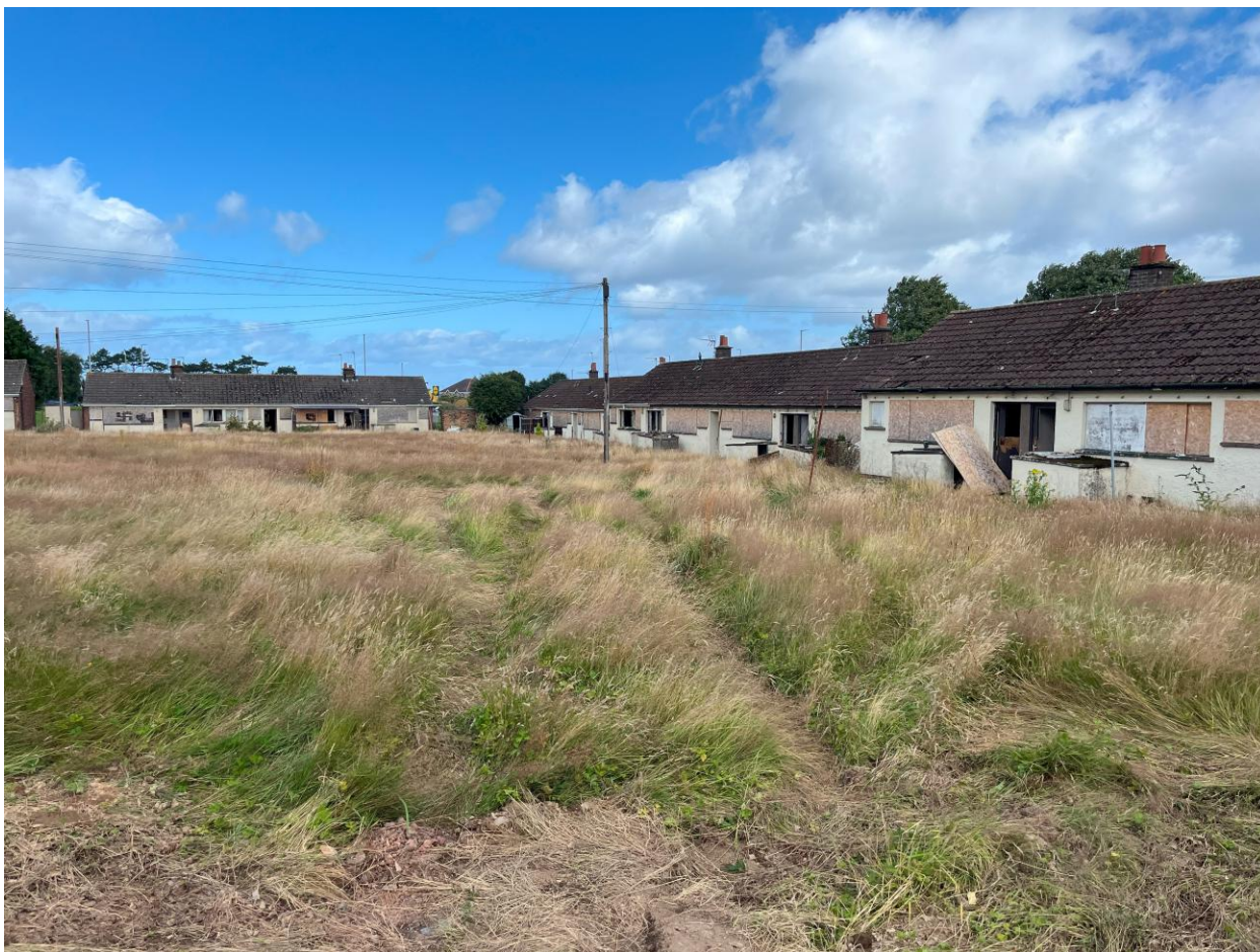
Photograph 7 – Central enclosed amenity area to the rear of dwellings
