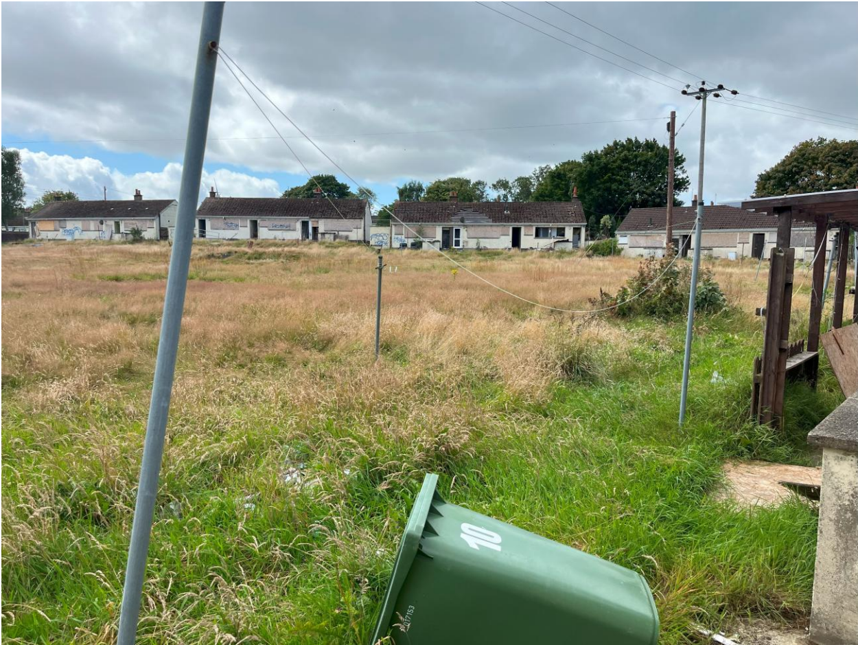
Photograph 8 – Central enclosed amenity area to the rear of dwellings
