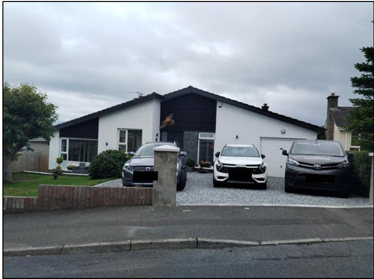
Figure 1. Front of the dwelling
