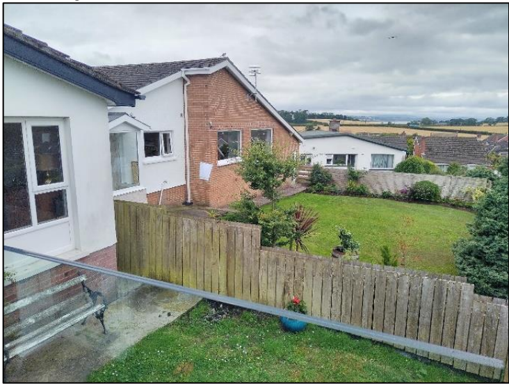
Figure 9. View from the terrace towards No.14 The Brae
