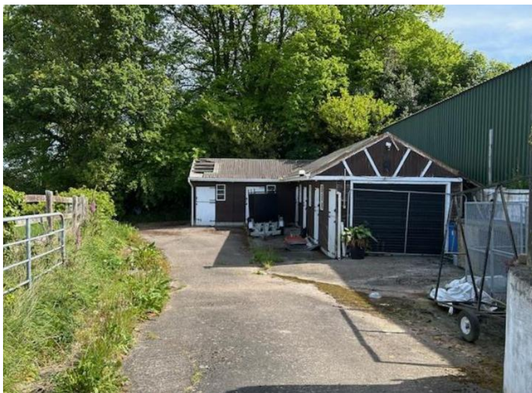
Garage/shed in yard to rear of dwelling
