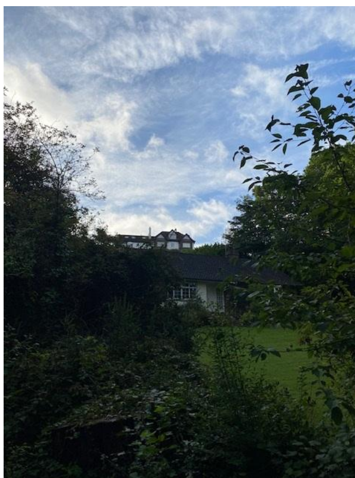
View of site and existing dwelling from 3 Woodlands Avenue
