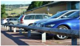
IMAGE - EXEMPLAR BOUNDARY TREATMENT Timber Knee Rail
