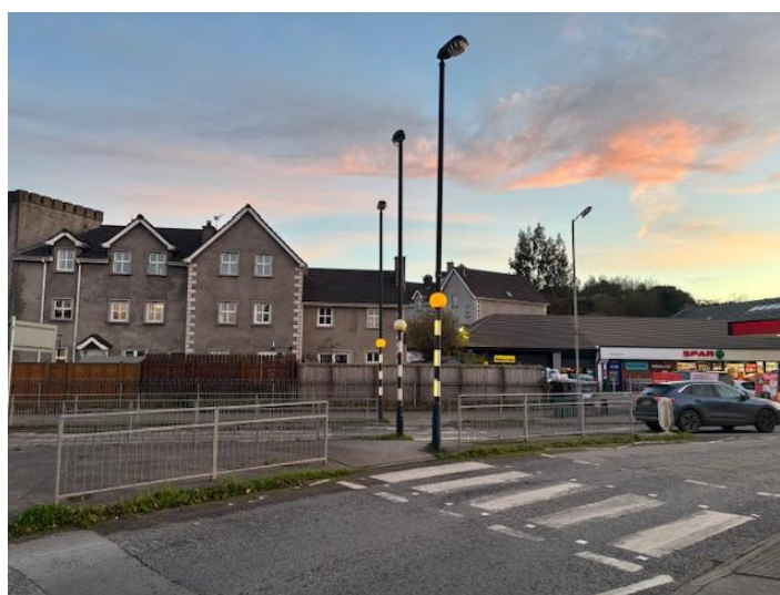
Figure 1 – Site viewed from Saintfield Road
