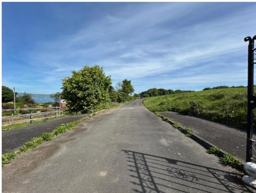
Existing access lane to 5 Woodlands Avenue
