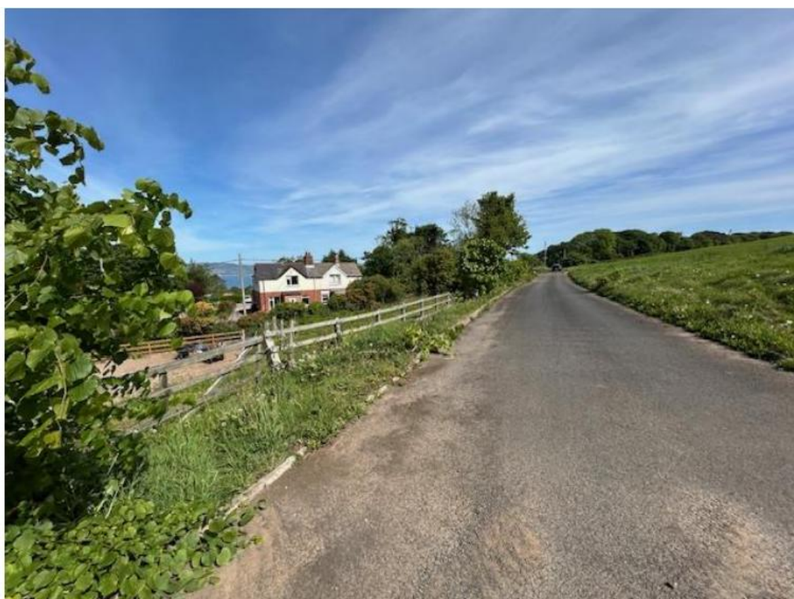
Existing access lane to 5 Woodlands Avenue and view towards The Cottages
