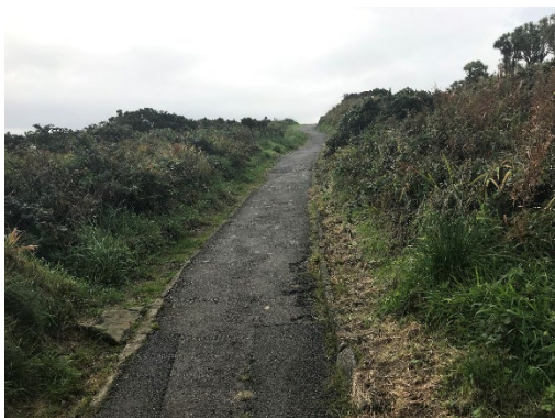
k) Poorly maintained, uneven, narrow path with steep gradient and broken edges.
