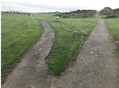
i) Narrow, poorly installed uneven paths with broken edges.
