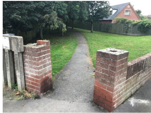
h) Narrow entrance, steep gradient and loose gravel path at Hunts Park entrance.
