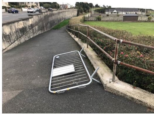
f) Steep Gradient and pedestrian obstruction on entrance path between Millisle Road and Putting Green site.
