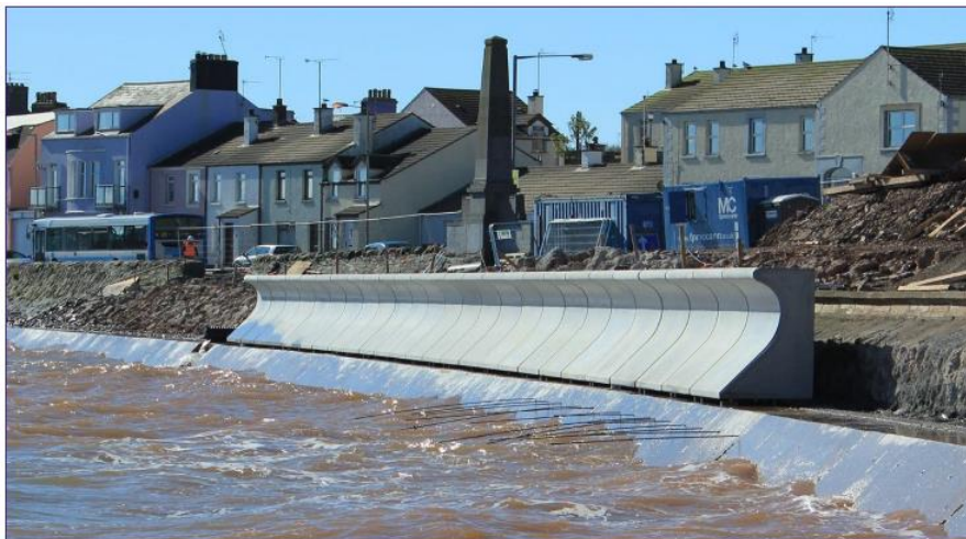
Image of existing recurve seawall at the outer Parade, west of lemons wharf, under construction in 2015, photo by Moore Concrete
