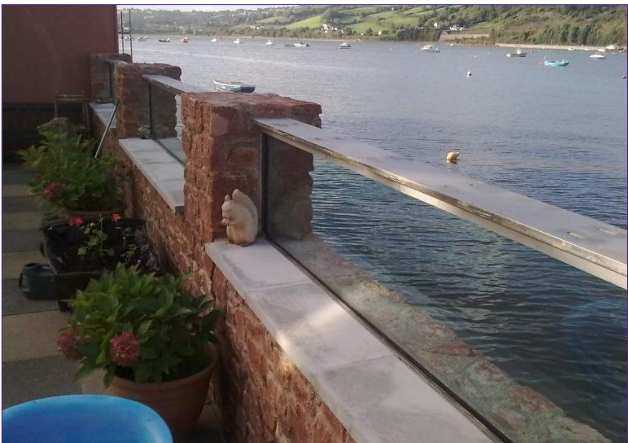
Figure 7-1: Image of Glass Flood Wall, by MM Engineering
