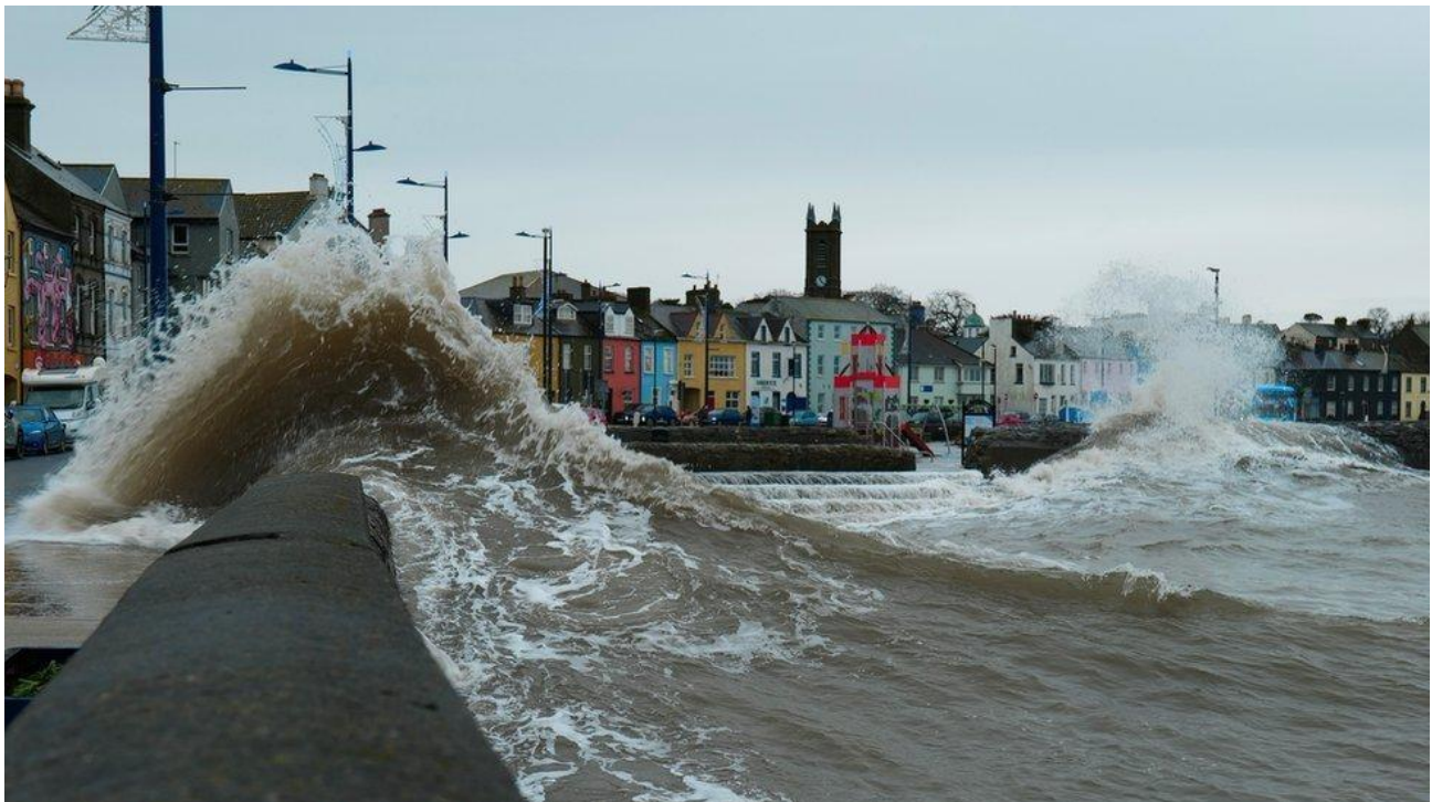
Figure 7-15: Example of oblique waves becoming "focused" and running along the existing sea defence east of Lemon's Wharf.
